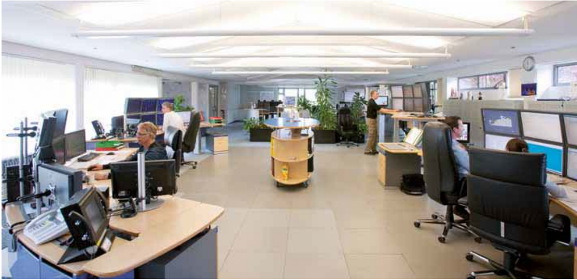
Schneiderkrug control centre
